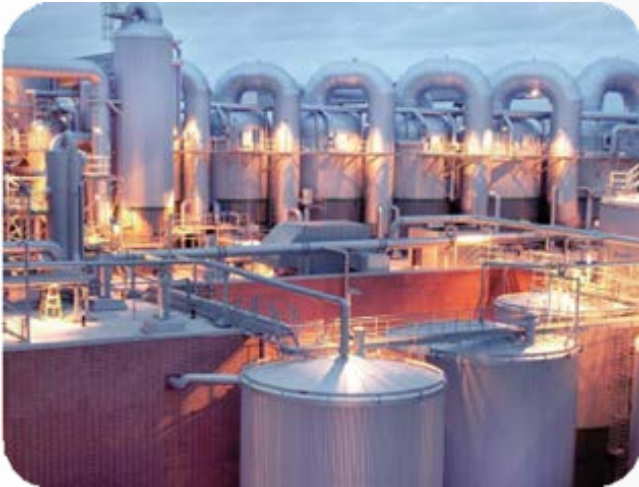
REFINERY, PETROCHEMICAL & CHEMICAL
